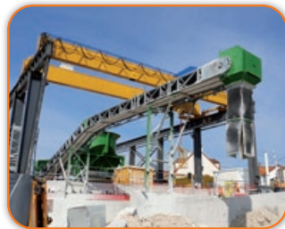
Travaux tunneliers Grand Paris Express
